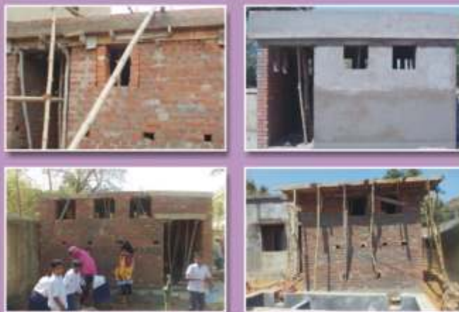
Pictures of current projects under construction
