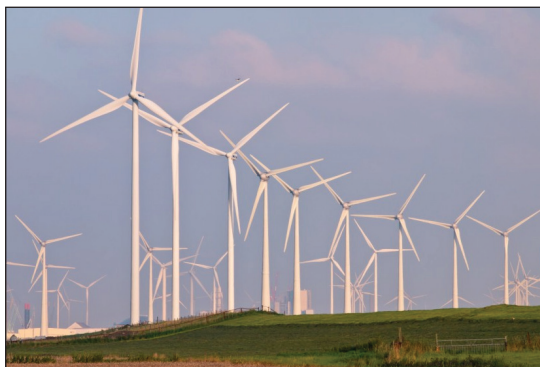
Wind Energy Project at Bothe, Maharashtra
