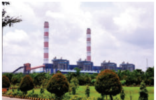
Jindal Power Plant
